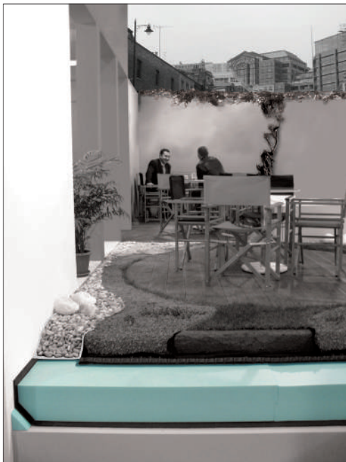
Composites of extensively greened roof. Roof is made of 20 cm thick FIBRANxps thermal insulation boards
